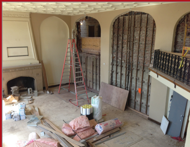
The entryway/foyer is being expanded and overhauled.
